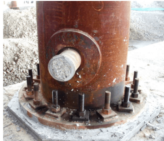
Figure 1: Concrete-filling of a composite HSS by pumping from the bottom
