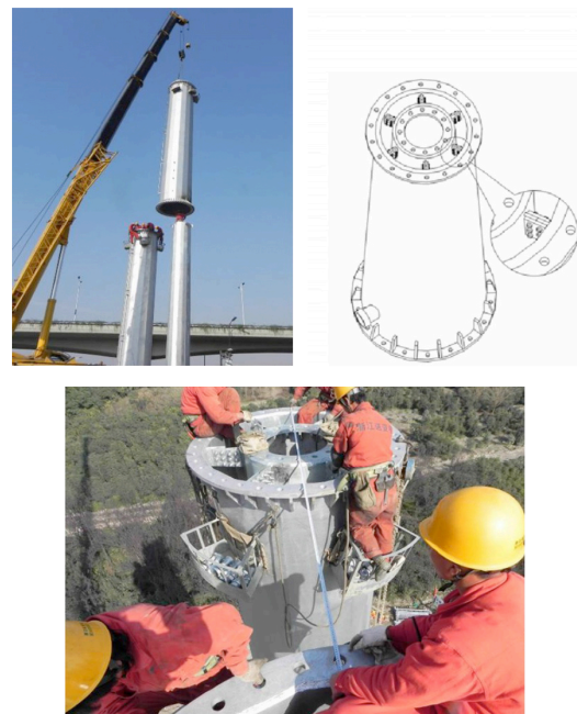
Figure 4: CFDST transmission line tower pole under construction in China (Li et al. 2012)
